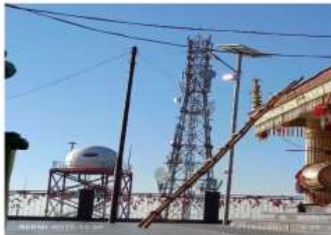
DOPPLER RADAR INSTALLED IN SURKUNDA DEVI
